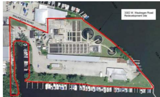
Figure 3.2. City of McHenry's former wastewater treatment plant.
