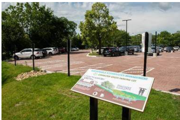
Parking lot with permeable pavers
